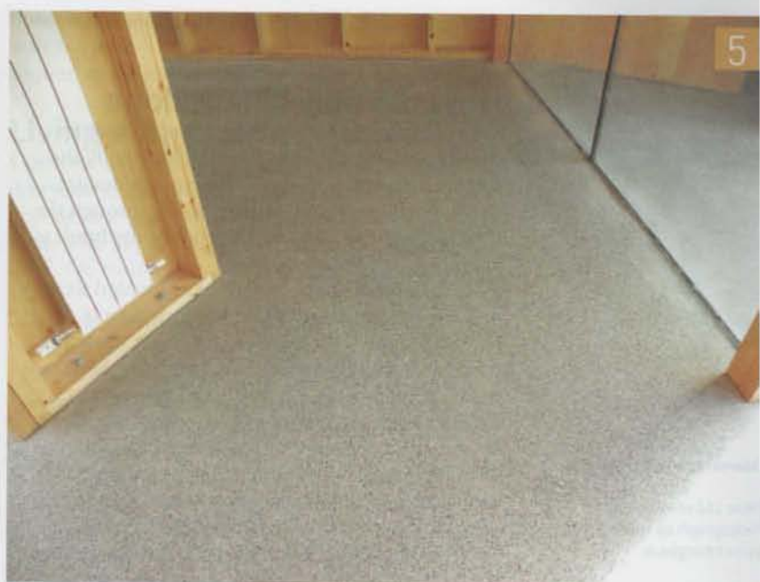
Stages to a new polished concrete floor: the concrete is poured (1), allowed to cure (2), ground down (3), impregnated with a hardener (4) and finally polished, sealed and buffed (5).
