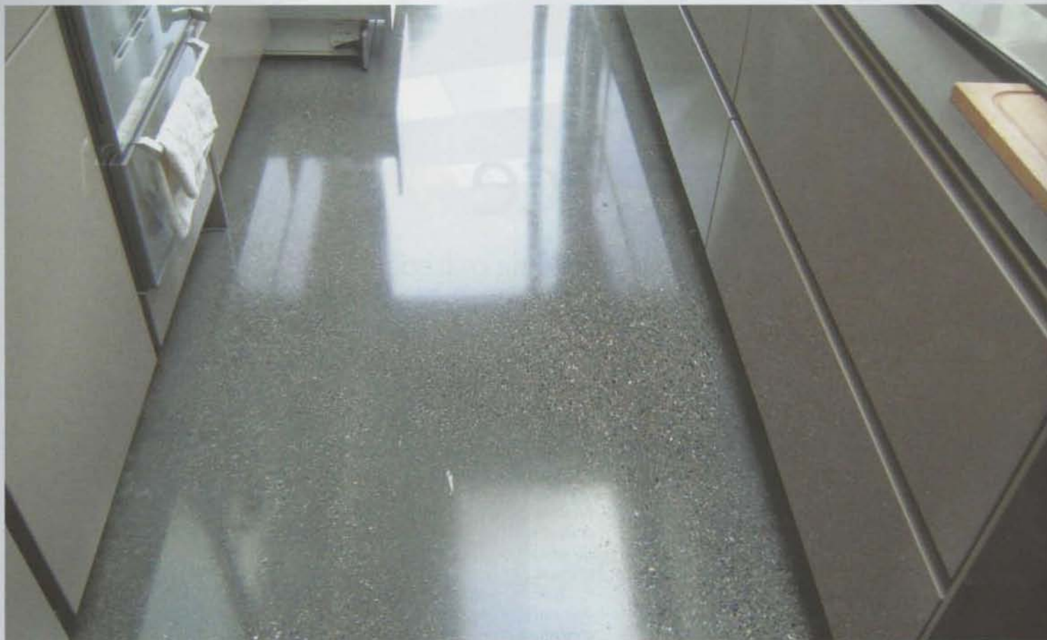
Concrete floor after polishing
